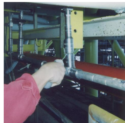
Checking during pressure test
