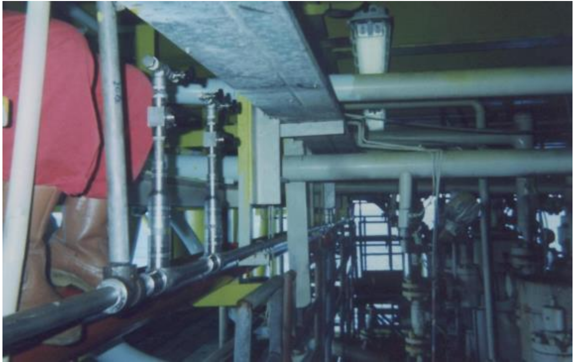
View of the completed line
