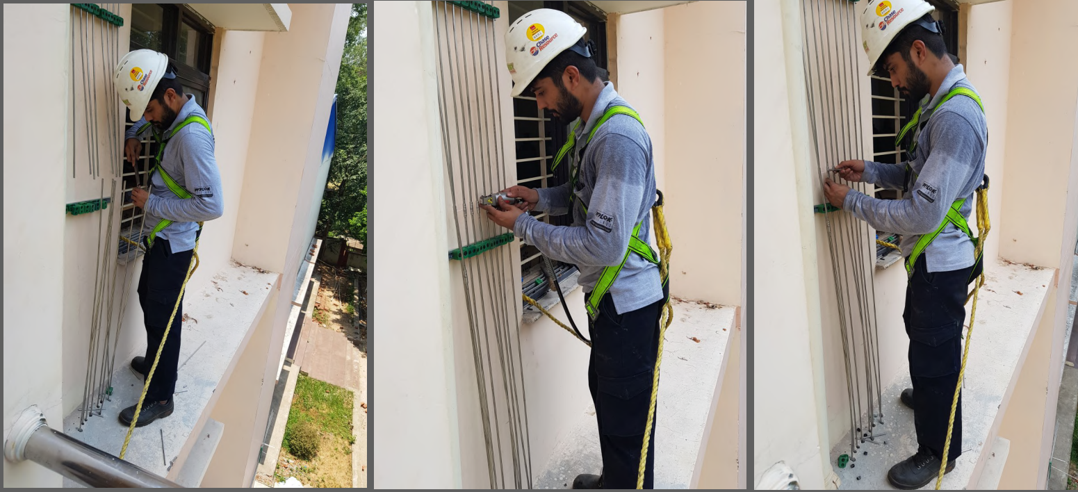
Above images showing the PYPLOK® installer installing PYPLOK® onto the tubing. As seen above, the installation in sequence- a) Check and prepare the tube end b) Crimp the fitting and c) Check and verify for proper crimp.
