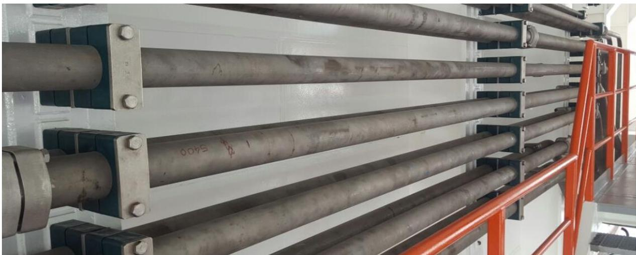
4. **Pressure Testing:** The installed pipes were Pressure tested to 1.5 x system working pressure by the customer installation team with hydraulic oil and was witnessed.
