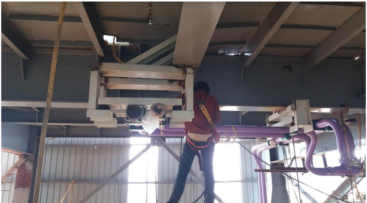
Hardline Installation
