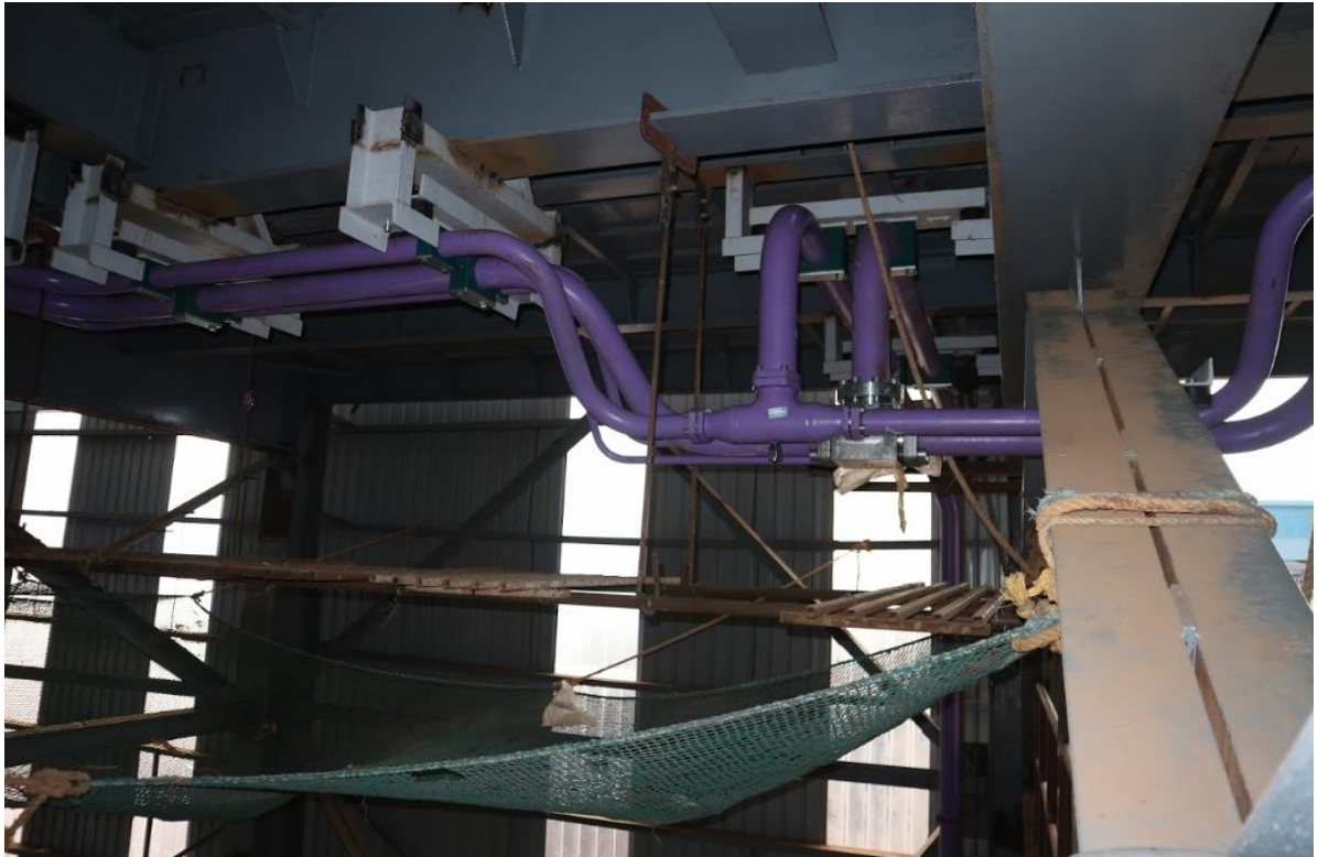
View of erected piping
