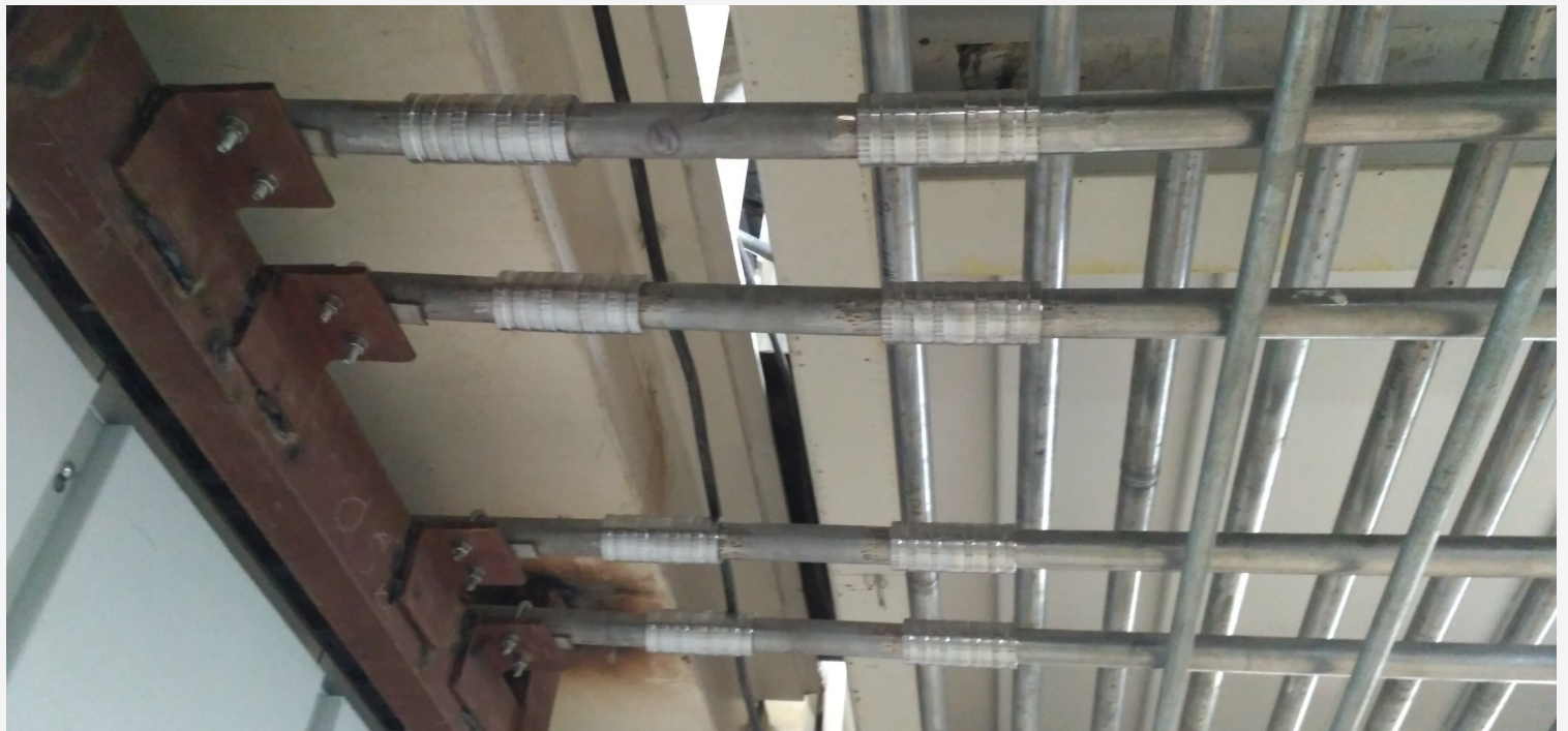
Pylok® fittings on the top pipe routing lines
