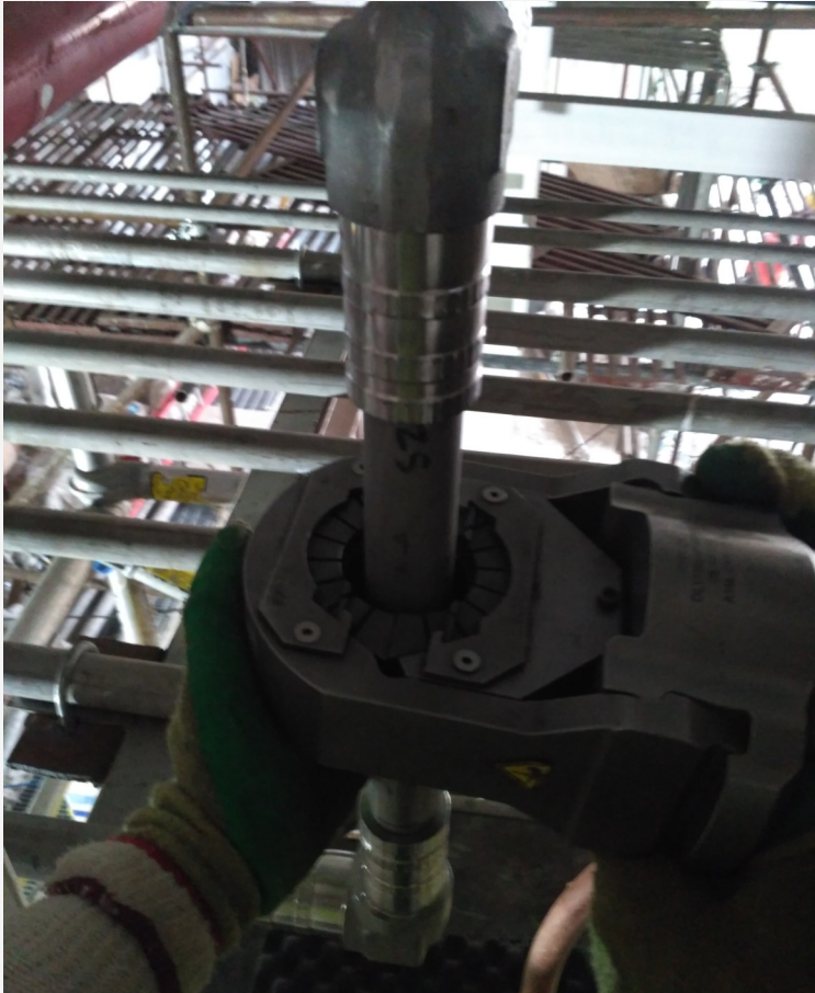
Pylok® Elbow installation
