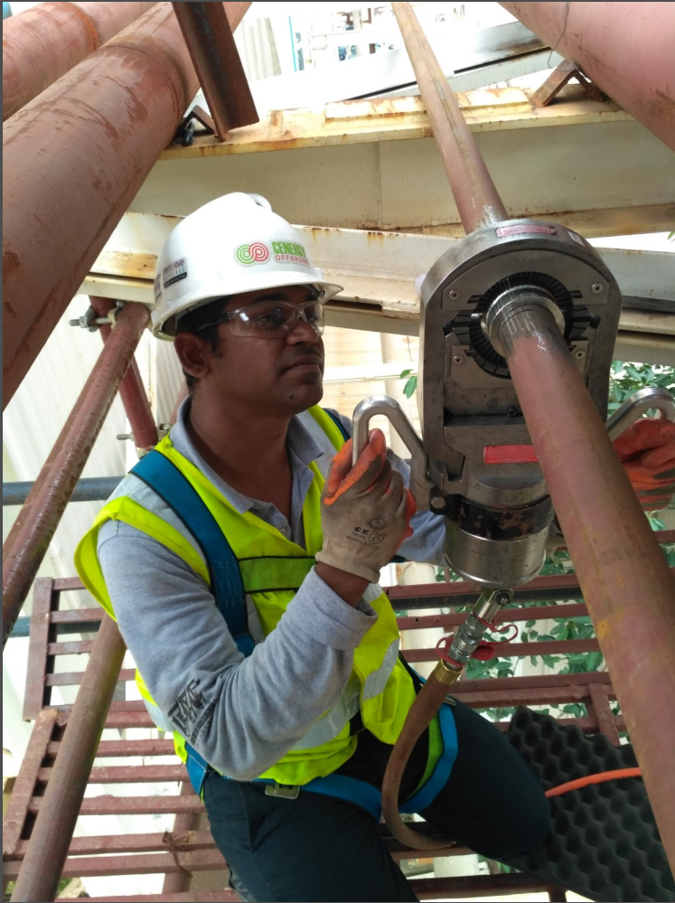
(left) CO technician crimping the Pylok® fitting (right) Fully crimped and inspected Pylok® elbows
