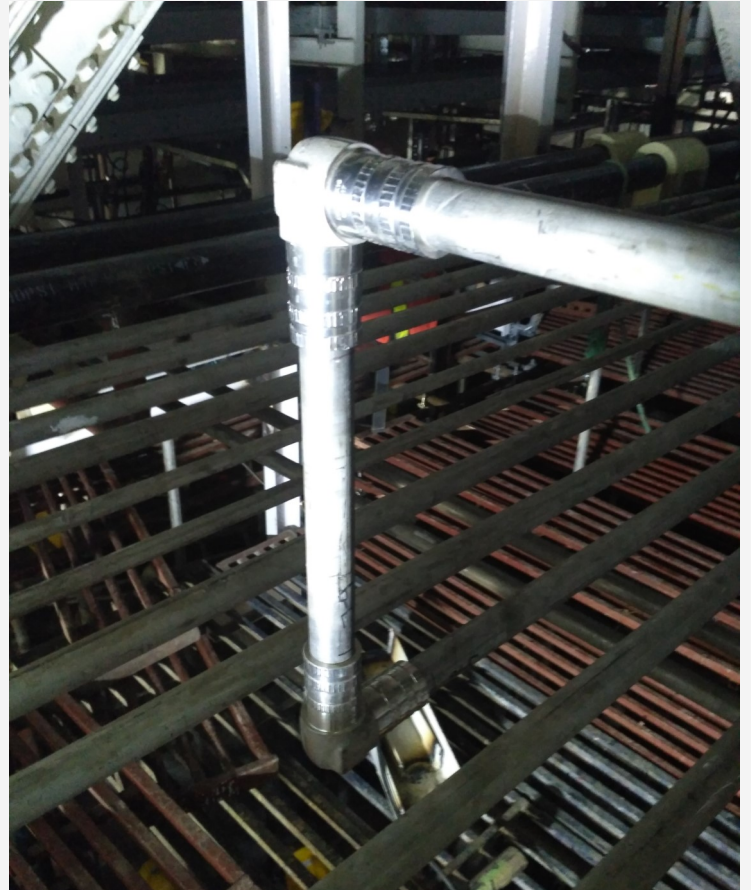
Pylok® Elbow installation
