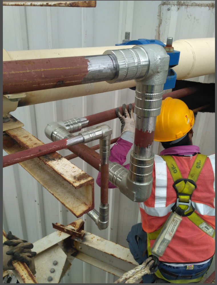
(left) CO technician crimping the Pylok® fitting (right) Fully crimped and inspected Pylok® elbows
