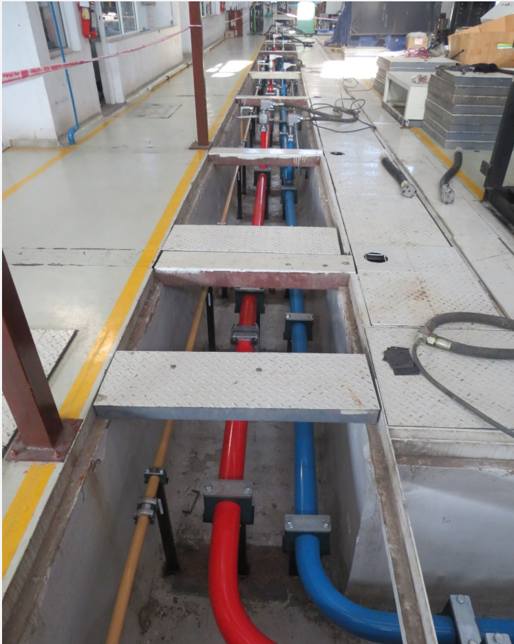
View of the hardline in a ring arrangement
