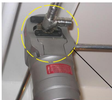
PYPLOK TOOL CRIMPING THE PYPLOK FITTING ON A WATER MIST LINE
