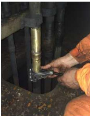
Cutting of Tube using Pneumatic Reciprocating Saw
