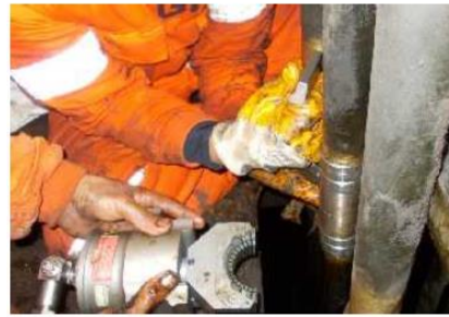
Crimping and inspection in any position
