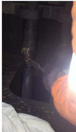
Removing Wrapped band by mechanical means
