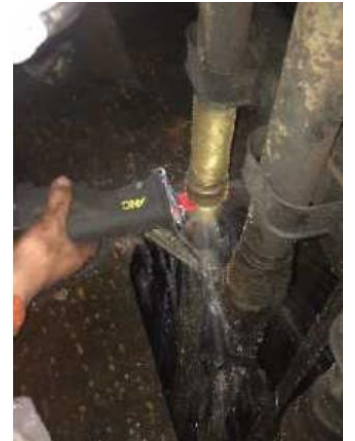
Cutting of Tube using Pneumatic Reciprocating Saw
