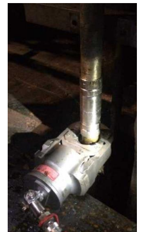
Crimping using Pyplok Power Unit Model 55 by means of pneumatic operated power pack XA11G
