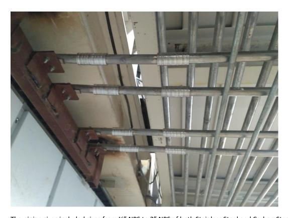
The piping sizes included sizes from  $\frac{1}{2}$ " NPS to 2" NPS of both Stainless Steel and Carbon Steel.
